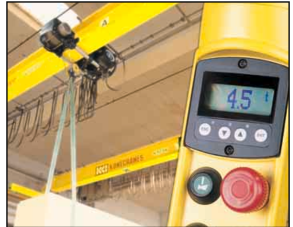
Continuous load control and overload protection for increased safety .
